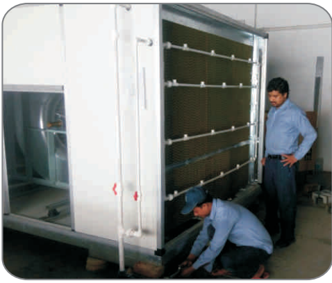
DOUBLE SKIN FLOOR MOUNTED AIR WASHER UNIT WITH SPRAY NOZZLES2
