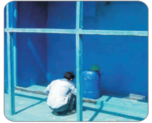
F R P WORK IN AIRWASHER CASING
