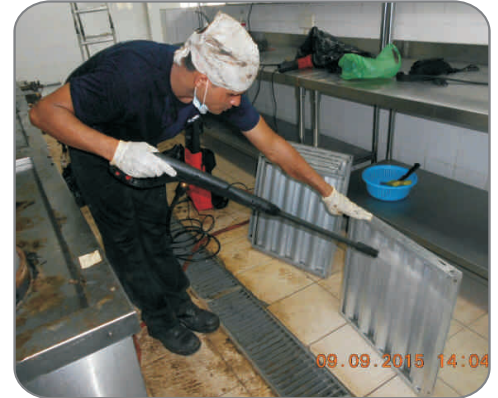
KITCHEN FILTERS CEILING
