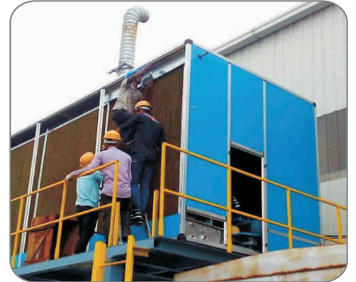
AIR WASHER ASSEMBLY ON SIT WORK
