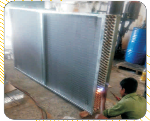
COOLING COIL REPAIR PROCEDURE
