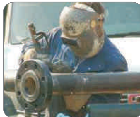
M/S PIPE WELDING WORK
